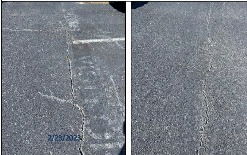
WBMS parking in main lot is cracking potential need for additional lot near cafeteria and art-wing – far right area
