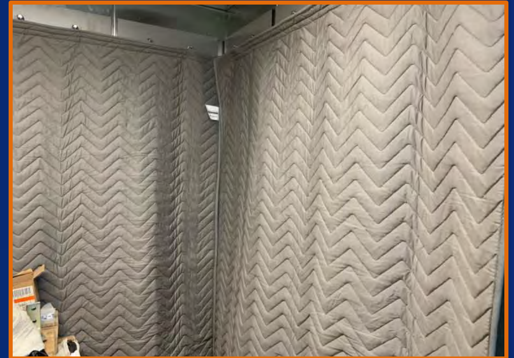
Quality Spotlight: Elevator Cab Installed and Protected
